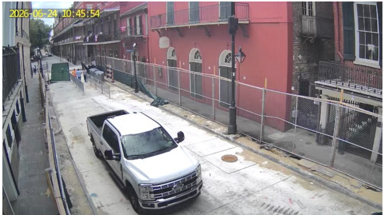
600 Block of St. Peters getting ready to shift work to sidewalk restoration
