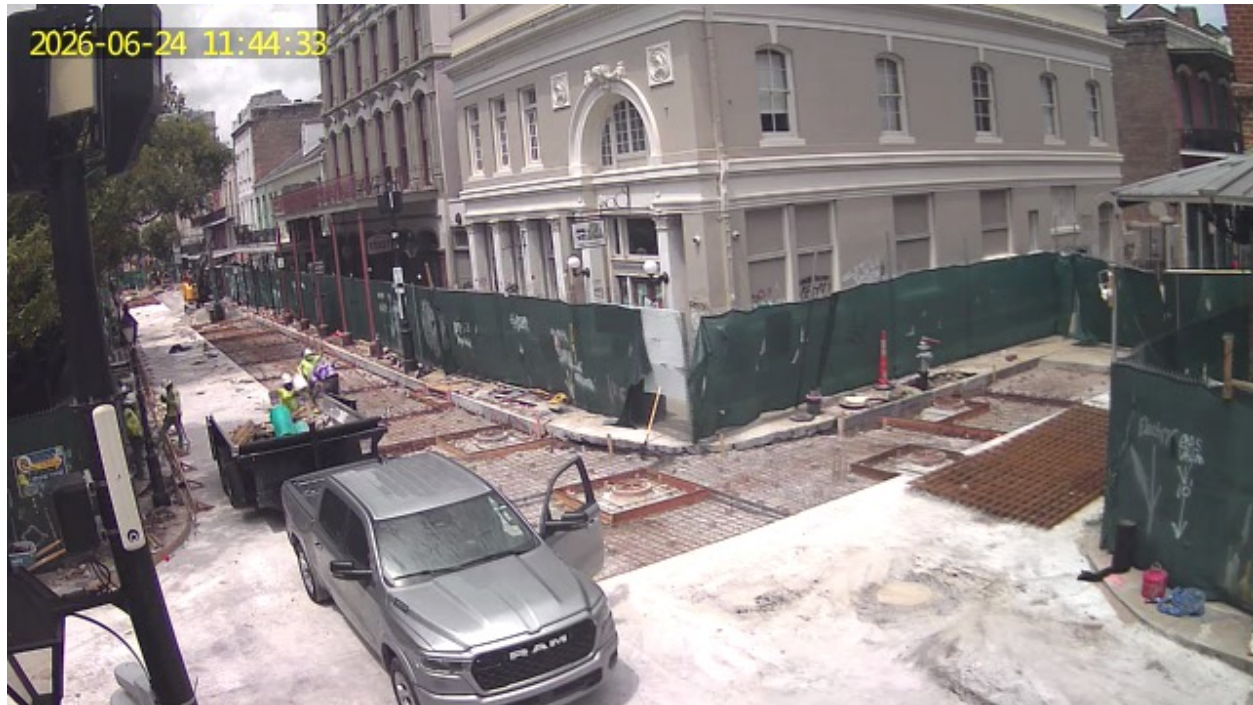
Decatur & Ursulines looking down the 1000 block of Decatur getting ready for final concrete pour
